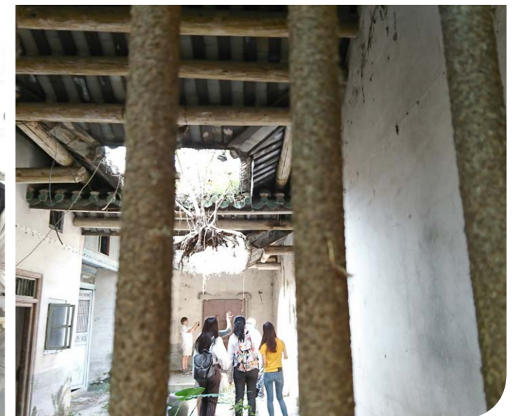
A group of students studying traditional Hakka roofing techniques and documenting the defects at the roof of Pun Uk Mansion. (Courtesy of Yumi Li Yeung-shin)
