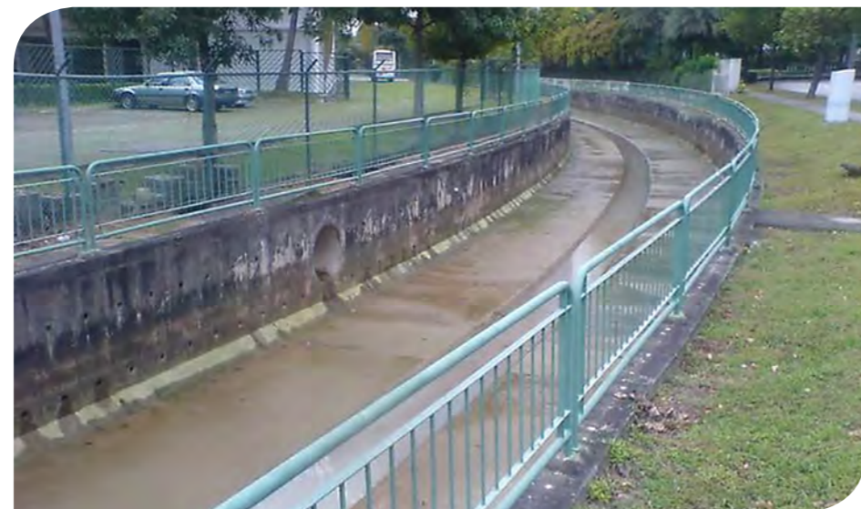
Conventional, non-sustainable, concreted-lined drain.
