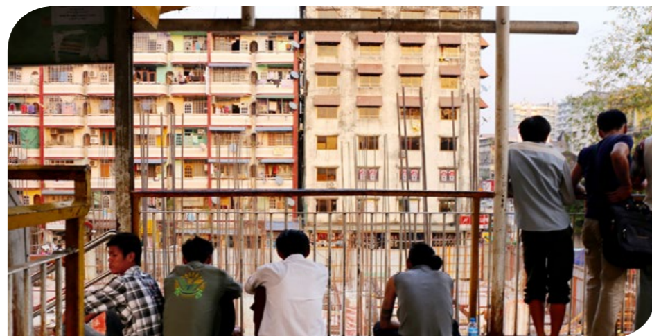
Construction underway in Yangon's historic district brings opportunities and threats.
