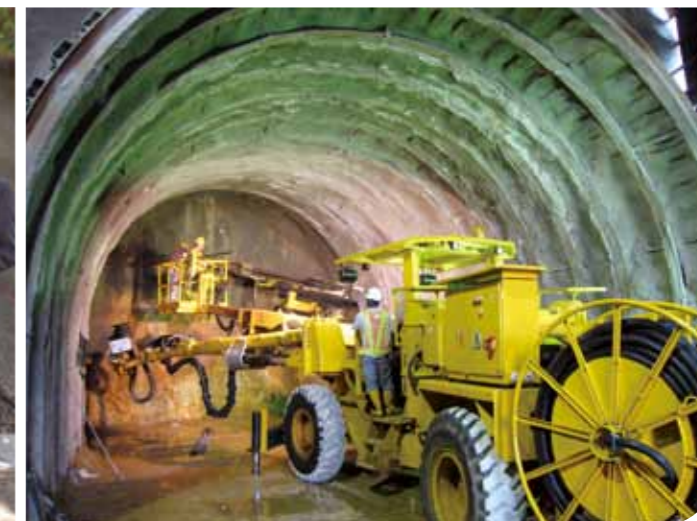
To minimise the disturbance caused to the environment and nearby residents, a non-explosive drill-and-break tunnelling method was used to house two saltwater reservoirs in a rock cavern.
