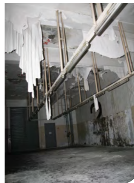
The exterior (top) and interior (bottom) of the historically significant Central Market, built in 1939, before being revitalised into a leisure-cum-recreational hub for public use. (Courtesy of Urban Renewal Authority)
